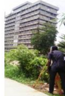
Fig. 7: Total Station at Reference Station C
